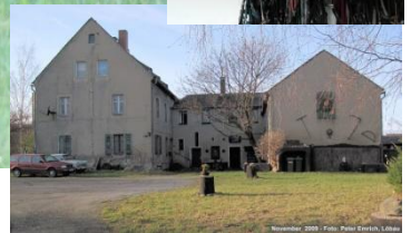
Damals: Deckstation in Löbau
